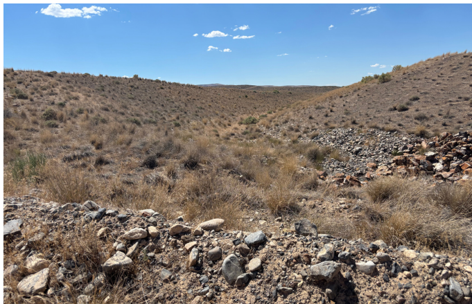
View of a drainage feature constructed at the toe of the reclaimed tailings facility
